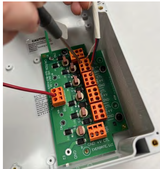
Figure 12: Install Source Cable Wire
