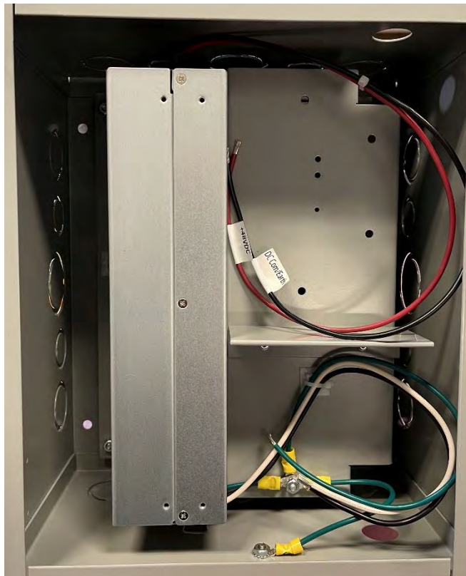
Figure 1: GPI Power Supply Module
